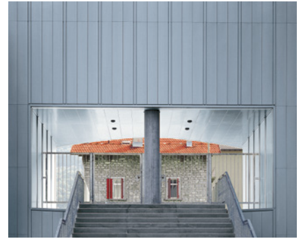
Telecom Giubiasco, Giubiasco, Schweiz
